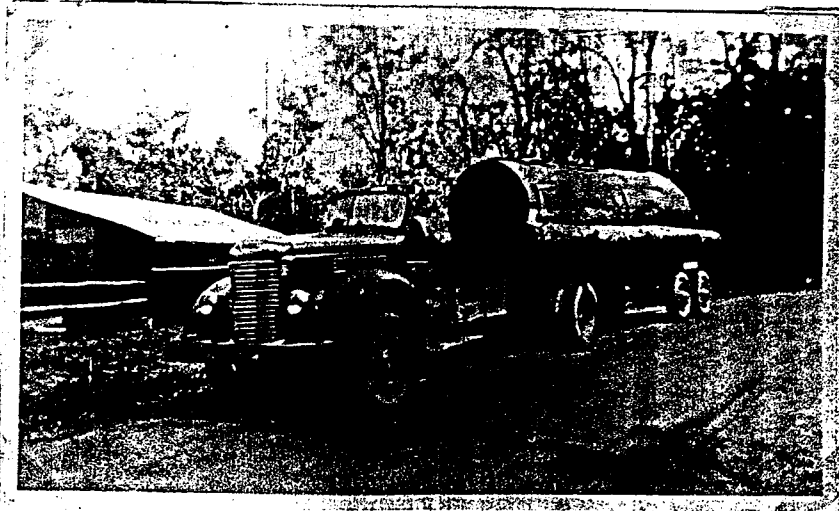
KS7 International Truck, 7-ton, tandem single wheel timber jinker
